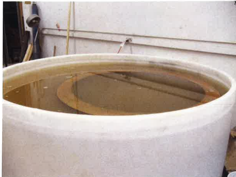
Figure 4. Saturation of manhole
