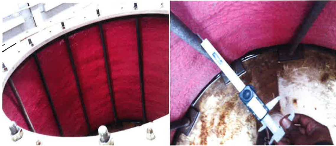
(a) View of the coating measurement
