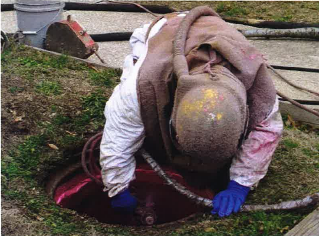
Figure 8. Applying initial barrier coat.
