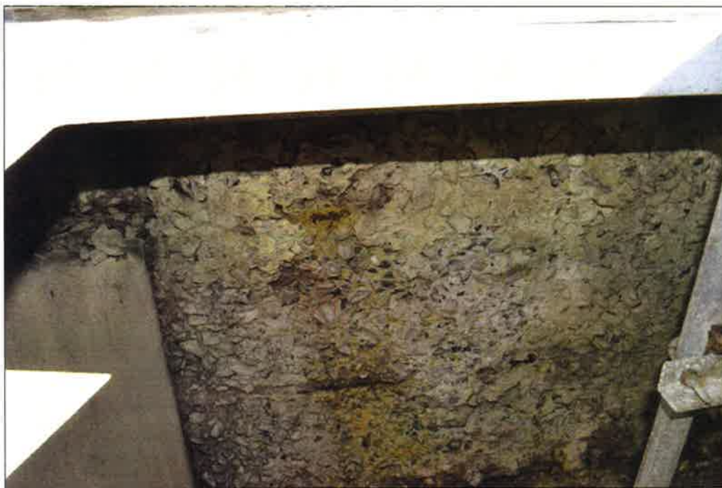
Figure 2. MICC deteriorated concrete and exposed rebar.
