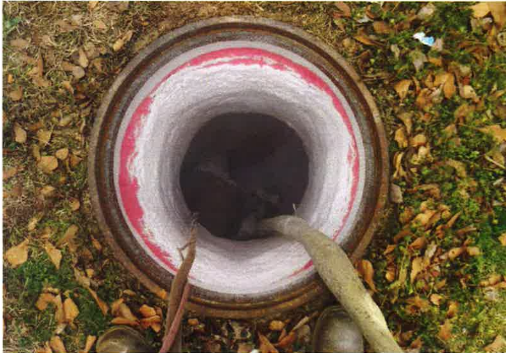
Figure 9. Applying foam over initial barrier coat.
