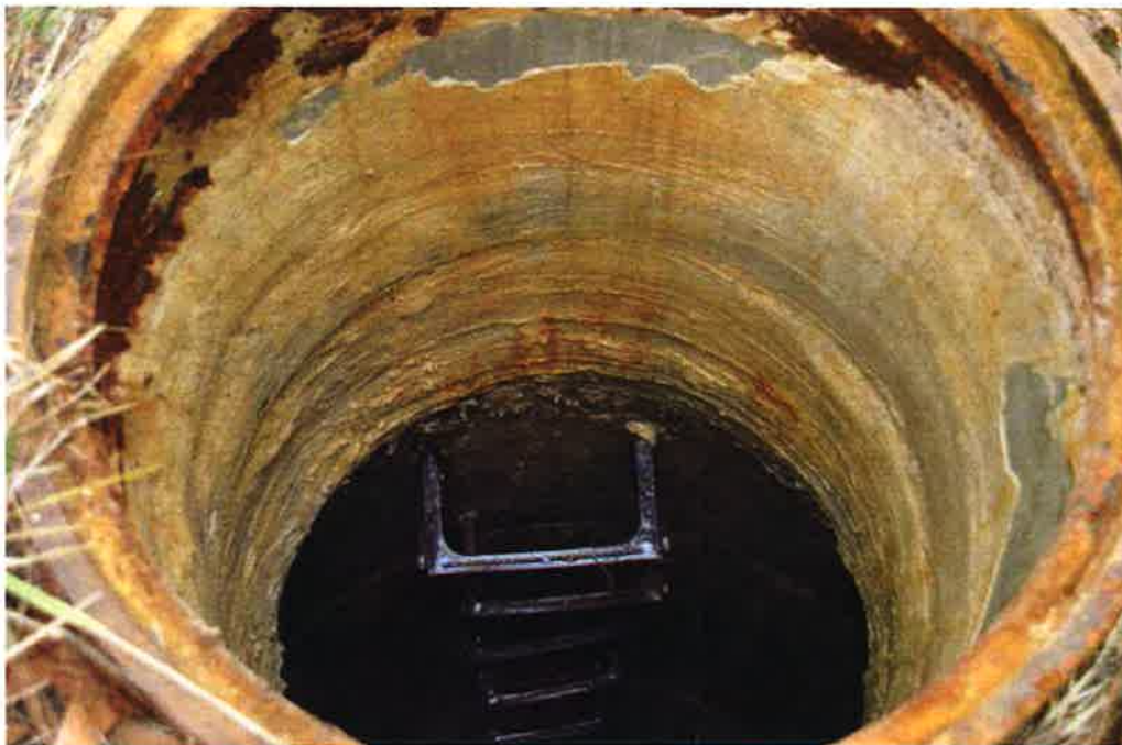
Figure 6. Ladder rungs to be removed.
