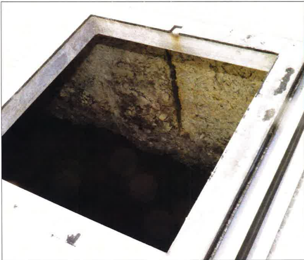
Figure 1. Example of MICC-deteriorated concrete in Fort Bragg system.
