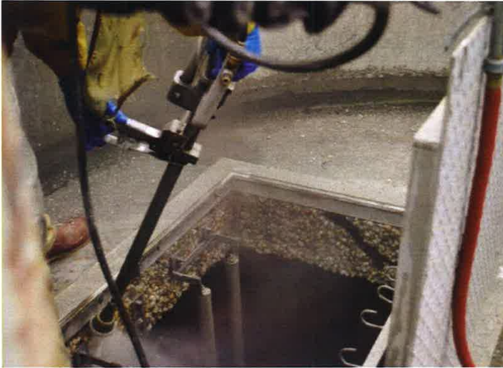
Figure 4. Hydro-blasting a lift station.
