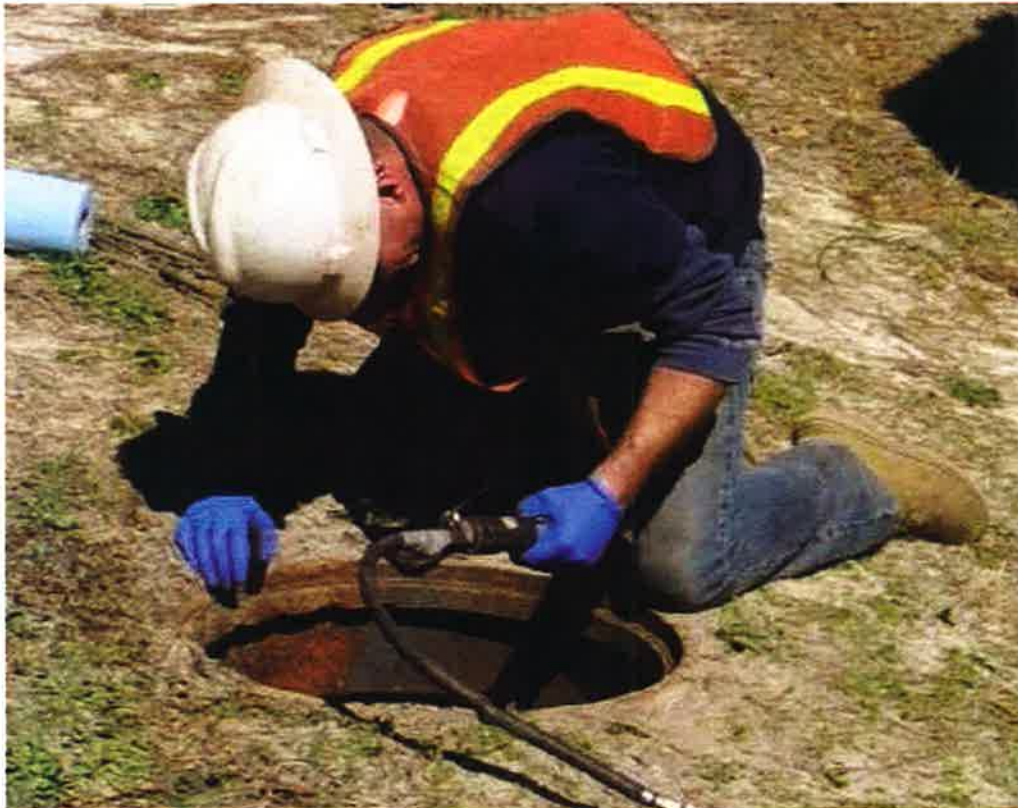
Figure 5. Rust removal of manhole entry ring.
